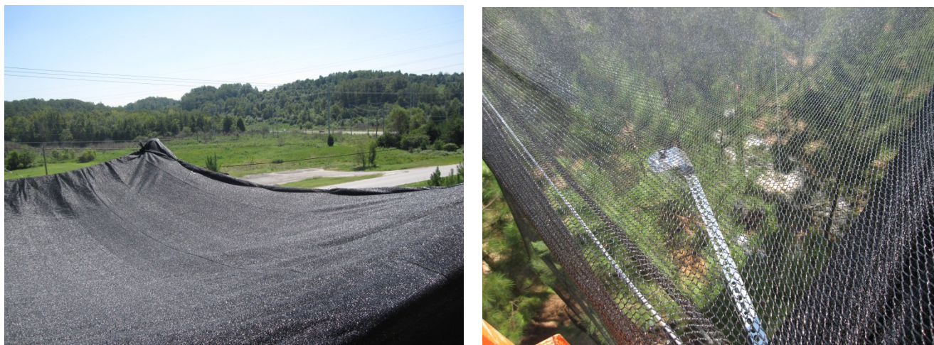
Figure 4. Completed shade treatment: (a) installed heavy shade cloth, (b) close up of heavy shade cloth.
