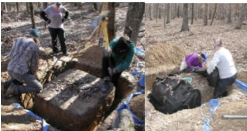
**Fig. 25. Trenching around soil chambers at MOFLUX, showing the excavation of a trench (left) and installation (right).**
